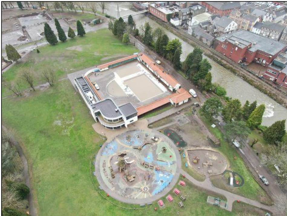
Figure 8: Image showing the flood damage to the National Lido of Wales at Ynysangharad Park following Storm Dennis (Image: Jonathan Lawrence/WalesOnline)
